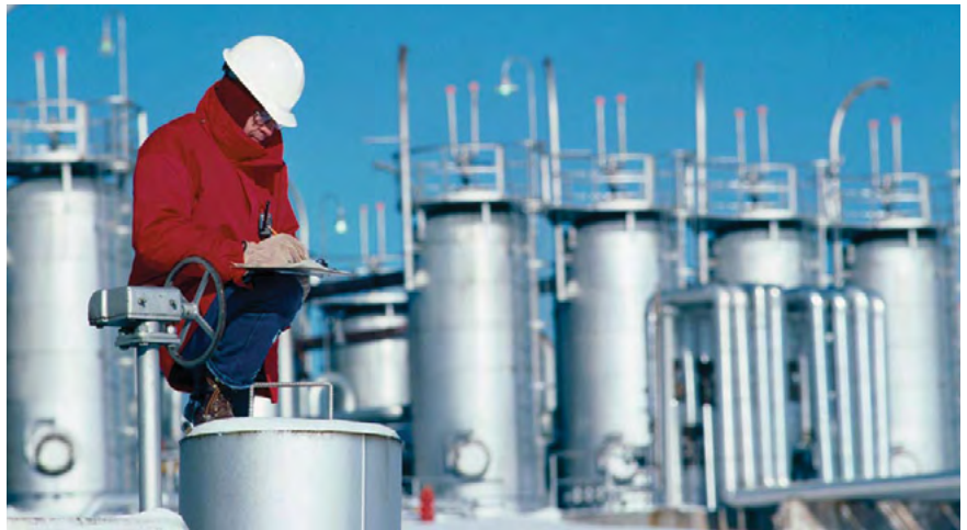
Planning on the ground at customer's factory for a first-time site assessment.
