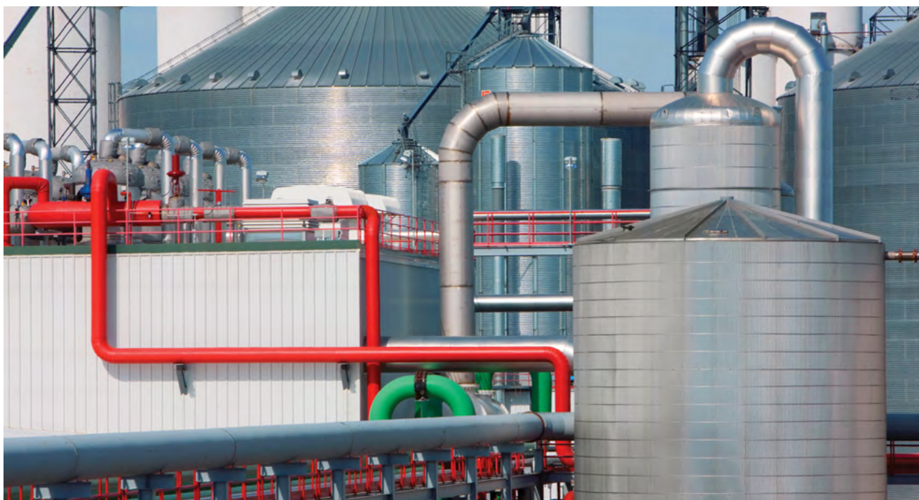
An example of a biorefinery similar to the one UPM-Kymmene is building in Leuna, Germany. Image: UPM-Kymmene.
