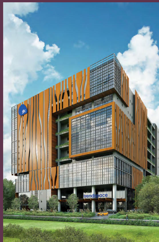
JTC's Trendspace, an eight-storey industrial building at Sungei Kadut, has received several awards, from design-related to safety awards.
