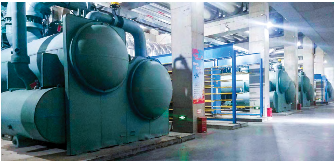
Figure 4: A geothermal heat-pump system provides heating and cooling in the low-carbon, Beijing Municipal Administrative Center.
