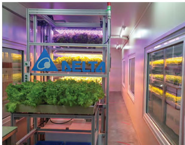
The interior of Delta's containerised plant factory at Punggol Digital District.
