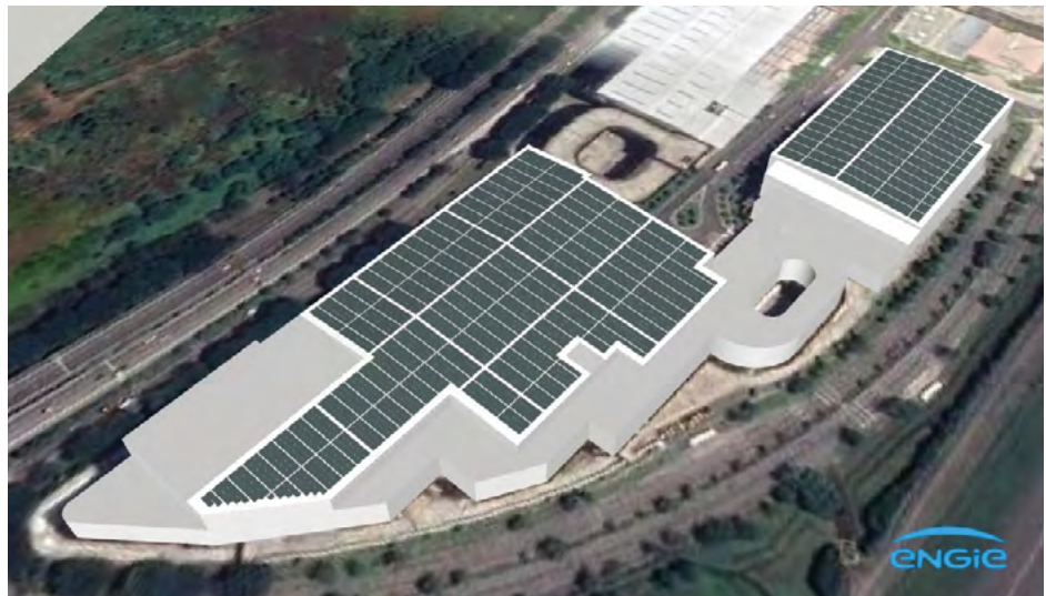
A mock-up of the ENGIE Renewable Energy Installation on DHL’s facility at a LOGOS estate in Singapore.
